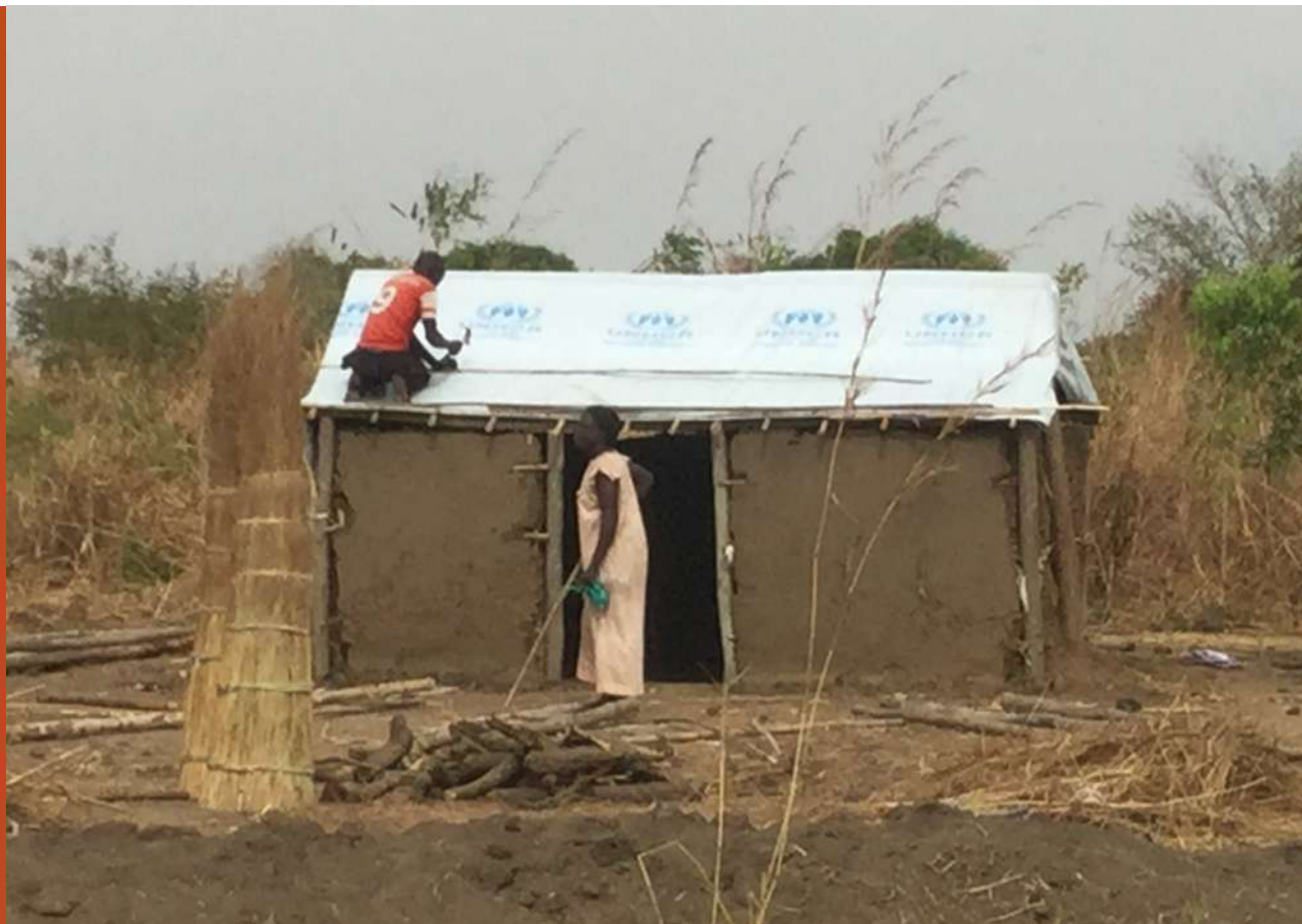
South Sudanese refugees constructing their homestead on land allocated to them by OPM in Adjumani: Photo Credit: RLP
